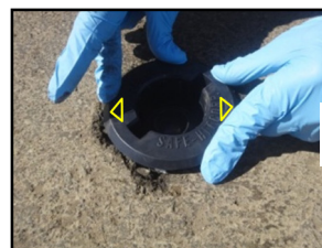
Place the SST Base into the hole with arrows facing the direction of traffic (lip is above ground).
