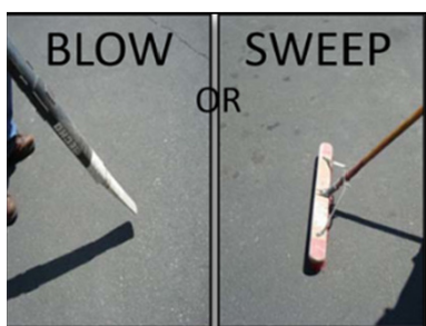
Sweep or blow area of debris
