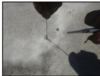
Use appropriate brush and compressed air to clear hole.
