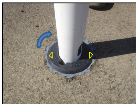
Place post in base and twist 1/8 turn clockwise to click into place (see note).
