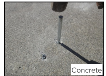
Set Drop-in Anchors with anchor setting tool.
