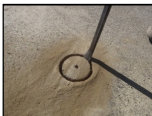
Pry out core section.
