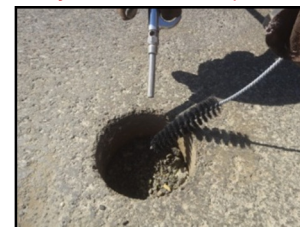
Brush and blow debris from hole.
