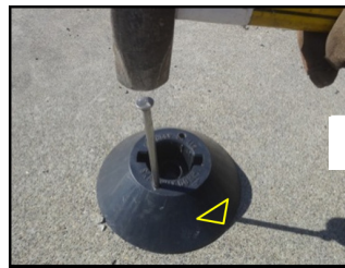
Use spike or 1/4" carbide drill to mark hole locations with arrows oriented in direction of traffic. Consult OSHA respiratory standards for crystalline silica exposure.
