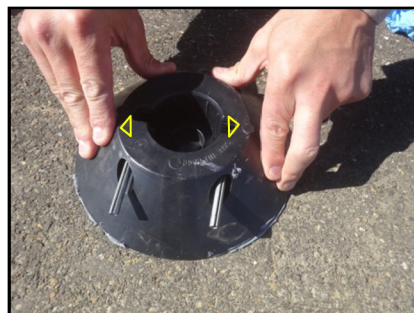
Place base on ground with the arrows facing the direction of traffic (both pins will be perpendicular to traffic).
