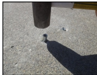
Place Anchors in holes and tap in with hammer.
