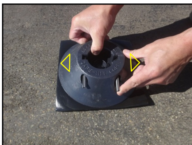
Place newly exposed side with arrows oriented with the direction of traffic.
