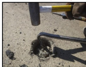
Chisel out remaining material from hole.
