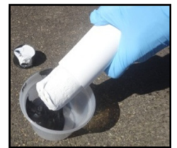
Use mixing stick to push epoxy into container. Thoroughly mix both parts to a solid gray consistency with no black or white streaks.
