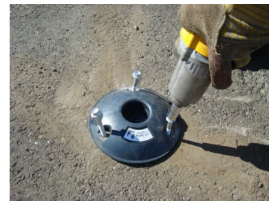
Step 6. Place the Base over the holes, and firmly tighten the screws.
