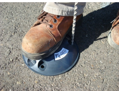
Step 3. Using the base as a template, mark the hole locations with a 3/8" drill bit.
