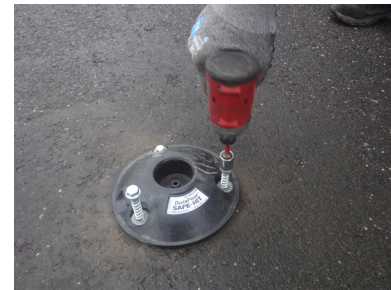
Step 5. Place the Base over the holes and firmly tighten the screws.
