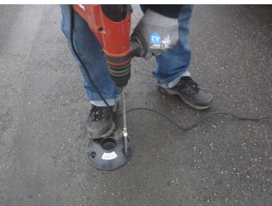
Step 3. Using the base as a template, drill holes 4" deep minimum.
