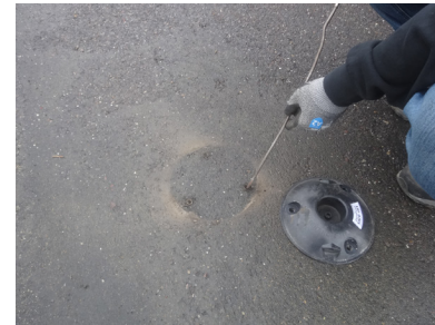
Step 4. Remove the base and blow or vacuum dust.
