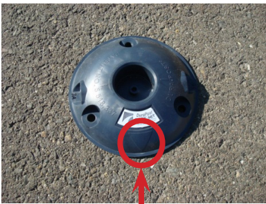
Step 2. Locate and mark Dura-Post® location(s). Position the base so that the arrow is pointing toward oncoming traffic.
