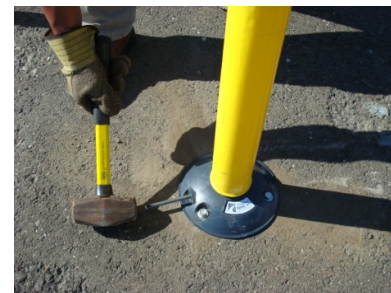
Step 7. Place the post with the holes aligned with the securing pin holes and secure with pin.
