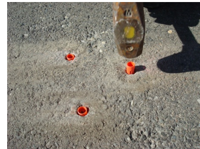
Step 5. Place the Nylon Expansion Anchors in the holes and tap with a hammer until they are flush with the road surface.
