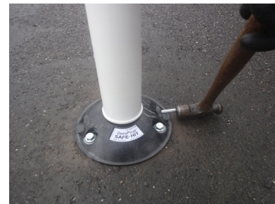
Step 6. Place the post with the holes aligned with the securing pin holes and secure with pin.
