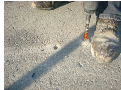
Step 4. Remove the base and drill 3/4" dia. holes a minimum of 5" deep.
