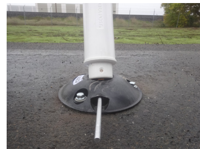
Step 5. Place the Base over the holes and firmly tighten the screws.
