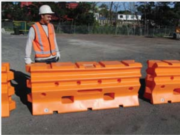
Figure 3: When setting out, ensure the configuration of the ends will fit together.
