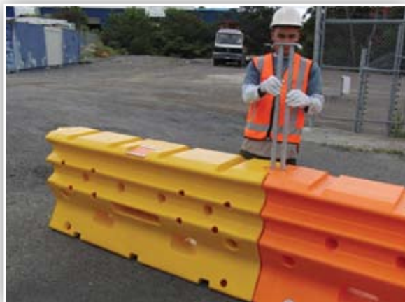
Figure 13: Once the units are aligned, the steel pin can be dropped into the alignment holes.
