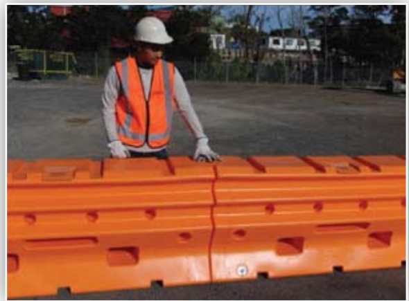
Figure 8: Check the steel pin has gone through the alignment holes.
