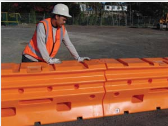
Figure 5: Units are pushed together to align the vertical holes
