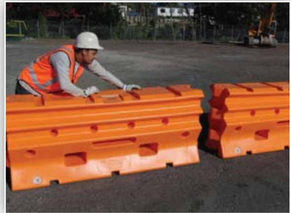
Figure 4: Sliding the units into position.
