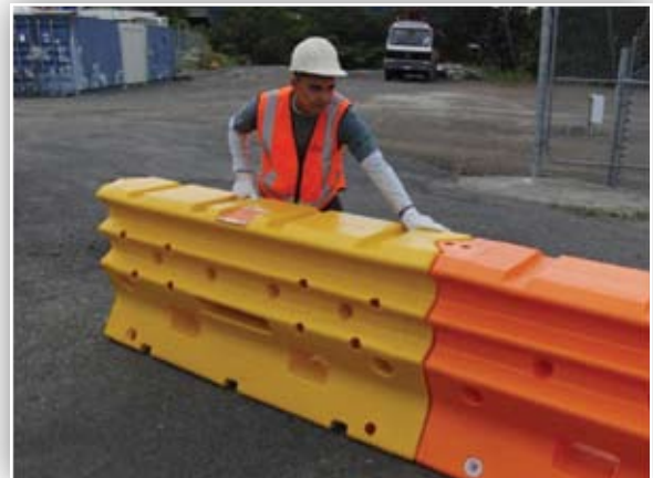
Figure 12: Slide the unit into position so that the vertical holes line up.
