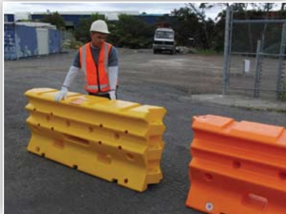
Figure 11: Position the end treatment unit so that the lugs line up with the end barrier unit.
