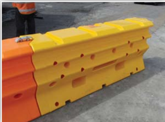
Installed End Treatment
