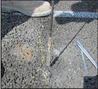
**Step 2:** Clean the holes using the pipe brush and compressed air. Ensure the holes are free of debris and moisture. Remove all dust and debris from the base site.
