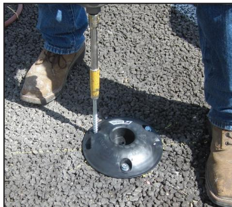
**Step 4:** Position the base over the holes and immediately place the anchors in the holes while the grout is still wet. Tighten screws until snug, but do not over tighten.
