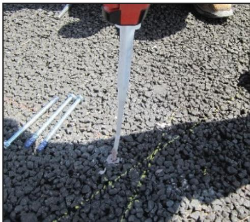
**Step 3:** Dispense grout into the holes. Starting with the dispensing tube at the bottom of the hole, work the dispensing tube tip up until the hole is filled to about 1/4" below grade.
