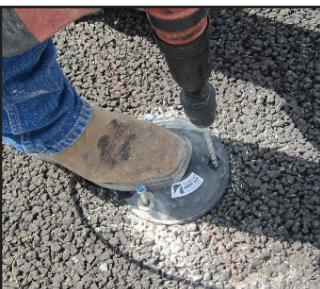
**Step 1:** Position the base so that the arrow is pointing towards oncoming traffic. Using the base as a template, drill 3/8" holes to a ground depth of 6" (+1/4", -0"). After the first hole is drilled, place a 3/8" bolt partially in the hole to help prevent the base from moving while drilling the next hole. Repeat drilling process for third hole.
