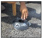
Step 5: Dispense grout into the holes. Starting with the dispensing tube at the bottom of the hole, work the dispensing tube tip up until the hole is filled to about 1/2" below grade. Place the assembled base in the holes filled with grout. Ensure the base is set firmly to the ground and not disturbed until the grout is fully cured.
