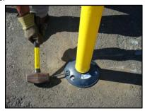
Step 7: Place the Dura-Post into the base socket and install the securing pin.
