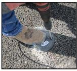
Step 1: Position the base so the arrow is pointing towards oncoming traffic. Using the base as a template, drill Ø3/8" starter holes approximately 1" deep. After the first hole is drilled, place Ø3/8" bolt in the hole to help prevent the base from moving while drilling the next hole.
