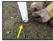
Step 5: Place the delineator tube on the anchor. Align holes to insert and secure selected fastener (tie wrap shown above).
