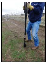
Step 3: Stand the driver tool upright, remove the pin at the top of the tool and then begin driving the anchor into the ground.
