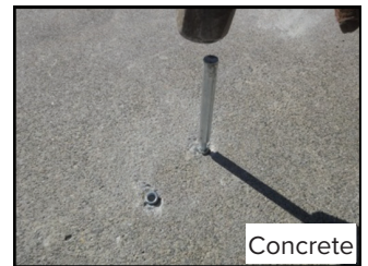
Set Drop-in Anchors with anchor setting tool.
