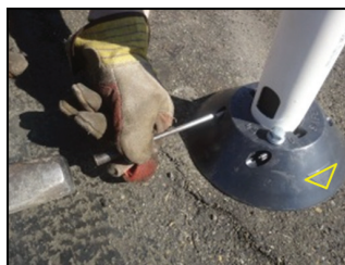
Complete driving the pins using a pin punch.
