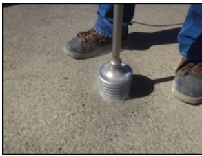
Drill 4" hole X 1 7/8" deep for SST Drill 4" hole X 2" deep for SLT
