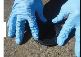
Place the SLT Base into the hole with arrows facing the direction of traffic (top surface is flush w/ ground).
