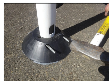
Allow the epoxy to set up, then place the post into the base and tap pins till flush with base (see note).
