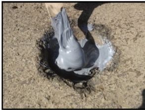
Drill 4" hole X 1 7/8" deep for SST Drill 4" hole X 2" deep for SLT
