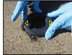
Place the SST Base into the hole with arrows facing the direction of traffic (lip is above ground).
