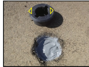
Apply epoxy evenly to the sides and bottom of the hole.
