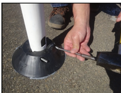
Use punch tool to seat pins into base
