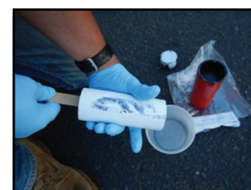
Use mixing stick to push epoxy into container. Thoroughly mix both parts to a solid gray consistency with no black or white streaks.
