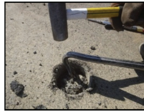
Chisel out remaining material from hole.
