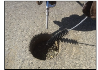
Brush and blow debris from hole.
