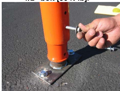
Step 9: Attach the 3/8" x 4" bolts with flat washers and locking nuts.
