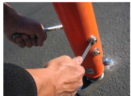
Step 10: Tighten the nuts until they are flush with the bolt end.
