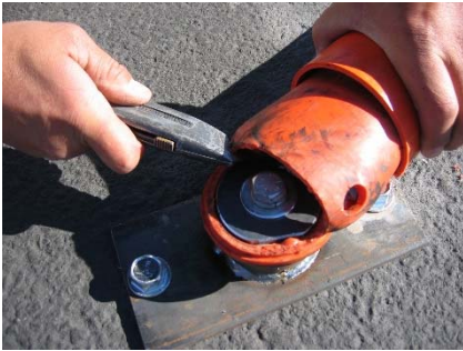
Step 1: Cut away old hinge tube.
