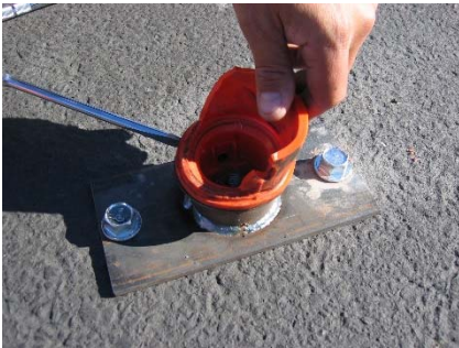
Step 4: Remove the old hinge section.
