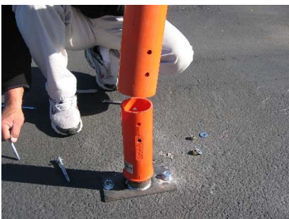
Step 8: Place the post on the hinge.
