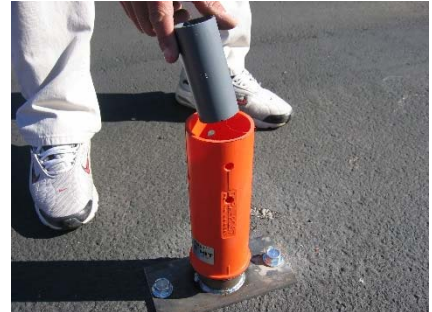
Step 7: Drop the inner tube into the hinge tube.
