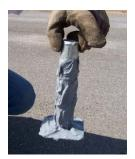
6: Insert the KonaPost® Anchor into the hole and press down firmly on the top plate until a bead of adhesive appears around the edge.
