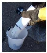
5: Apply a generous amount of adhesive to outside diameter and the underside of top plate of the KonaPost® Anchor (PN 603667).
